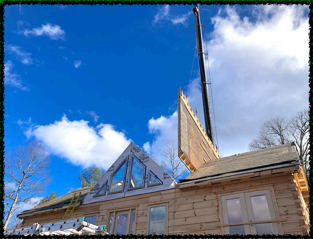
The BlueRidge Log Cabins crane crew artfully setting the roof peak on the Phillips new home in December. The home was fully dried in before our BRL community experienced a week of snowfall. The Irving home and the Phillips home are scheduled for completion in the first portion of 2025.
